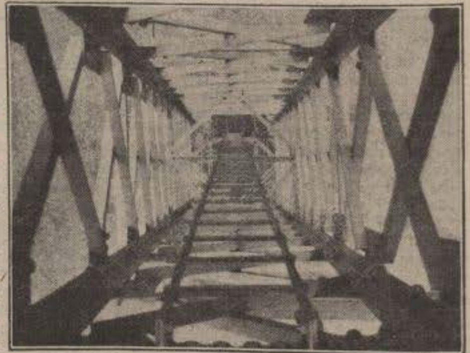
Listeners who have 'no head for heights' should not stare too long at this unusual photograph, which shows, from the top, the inside of one of the giant masts at Brookman's Park.
